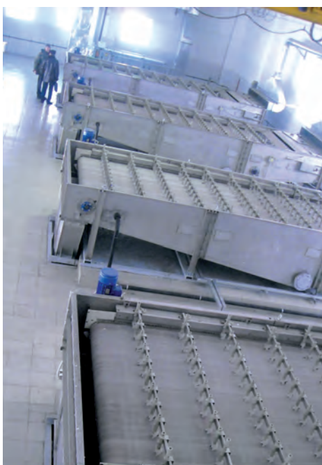
Sludge thickeners
