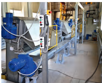
Mechanical treatment package based on screens RKE and screw conveyor KVE
